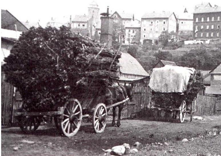
*Fig. 5. Carts bringing bark to a tannery in the city of Siegen in the early twentieth century. This is the type of cart Simon Dreisbach would have used for the transport of bark to Cologne in the spring of 1726. The wheels are oversized, not only for stability, but so that the carter could grasp the spokes to help move the cart forward where the ground was soft, or on inclines.<sup>8</sup>*
